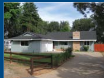
Structure completely restored
