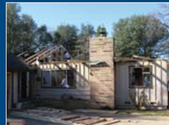
Rebuilding the structure
