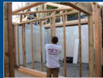
All fire & smoke damage removed
